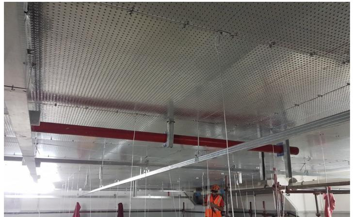
Promat Durasteel® is unparalleled as a high security fire protection board. The load-bearing, non-combustible A1-rated material – tested and certified to both cellulosic and hydrocarbon fire curves, is a market leader in barrier and ceiling systems, serving a wide range of industries as heat shields, blast and fire walls, and heavy duty enclosures.
